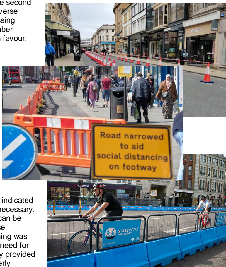
Pavement widening in Harrogate and London. Survey comments highlighted the risks these measures posed to cyclists, their impact on traffic, lack of permeability for pedestrians and their lack of use.
